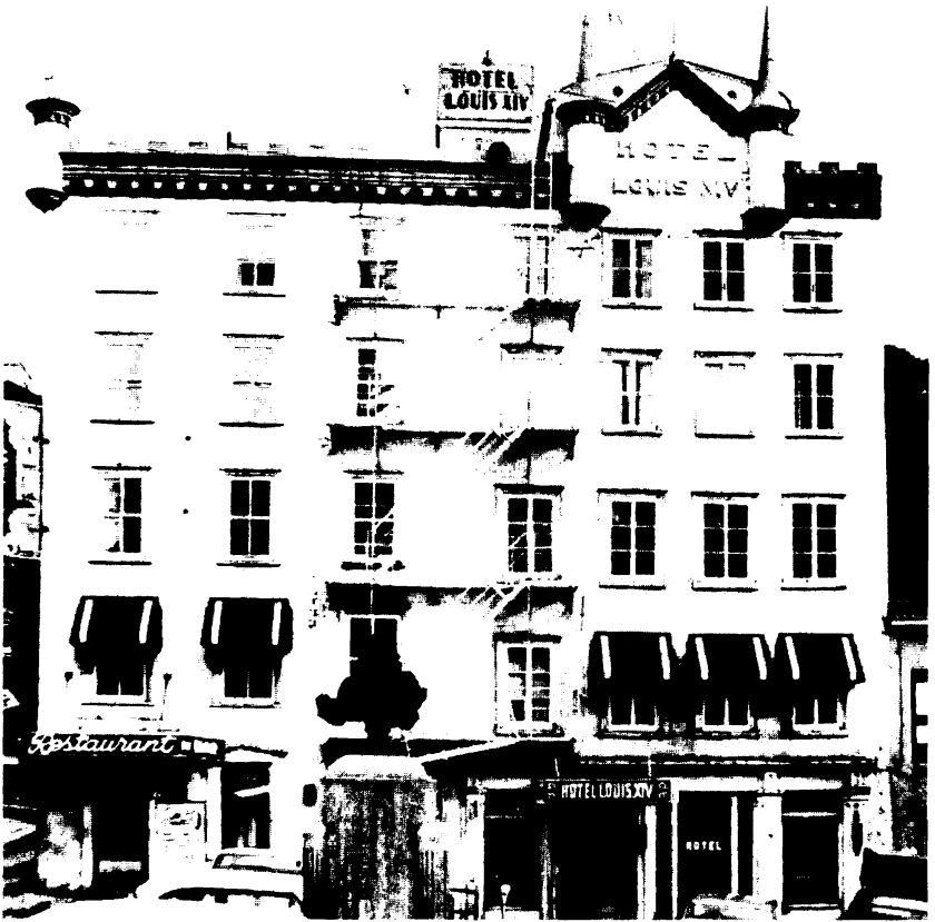
Hotel Louis XIV, Quebec City, in 1966. Note pattern of windows on second and third floors (courtesy of the Ministère des Relations internationales and the Ministère des Affaires culturelles, Quebec).
