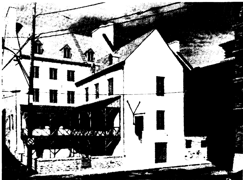
La Maison Leber, Place Royale, after its restoration (courtesy of the Ministère des Relations internationales and the Ministère des Affaires culturelles, Quebec).
